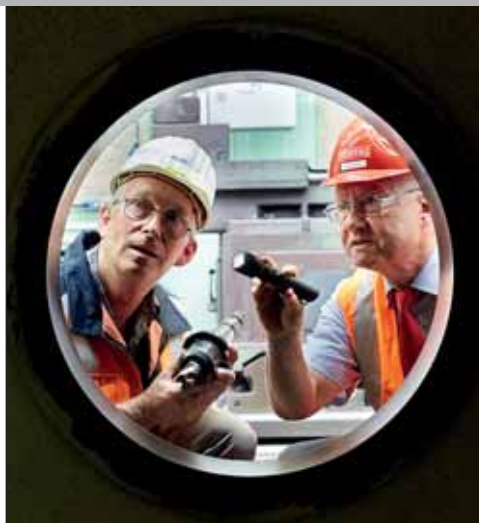
Teamwork at its finest: Willi Spelter (RWE) and Norbert Ophüls (DST) work closely together during a retrofit
