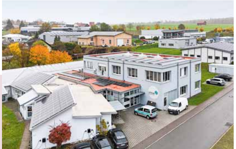
Based in Neuhausen ob Eck, Germany, the company employs around 100 people and has a modern machine park.
